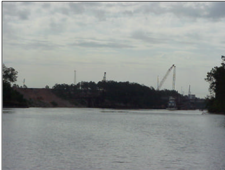
Photo 1. Bernard Bayou at Entrance to Industrial Seaway
