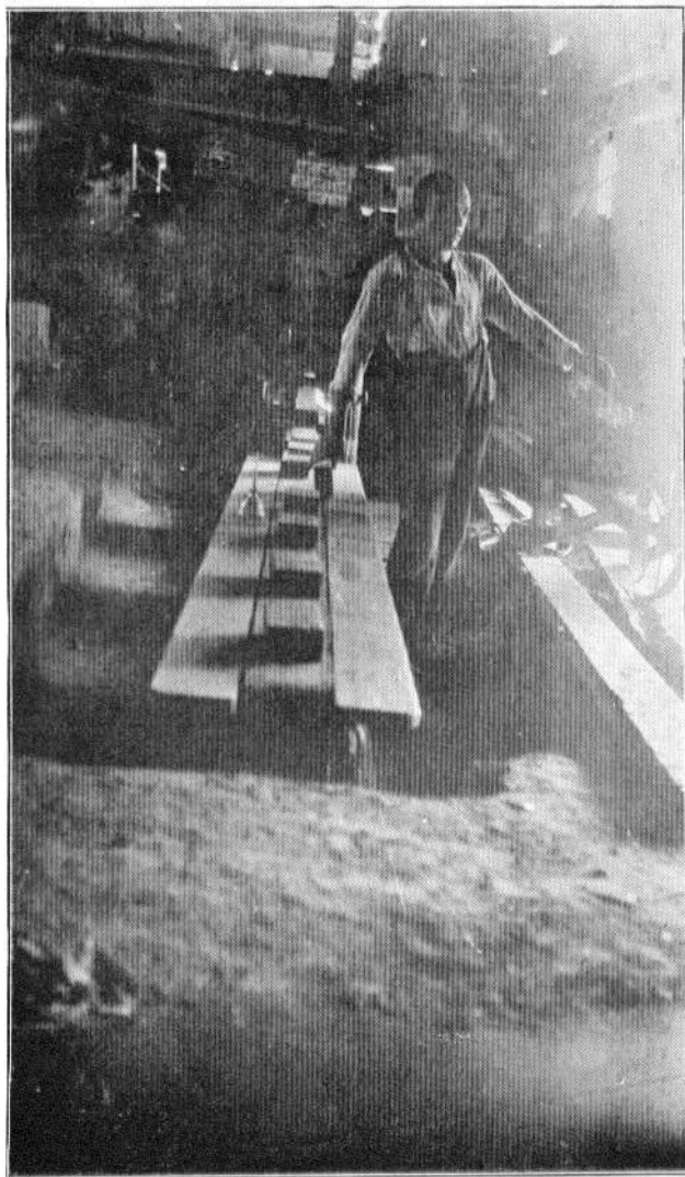
TAKING BRICK FROM OFF-BEARING BELT OF AN END-CUT MACHINE.
