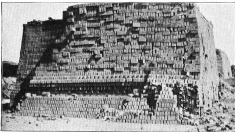
A. BURNED BRICK IN A SCOVE KILN; GOOD BURN.
