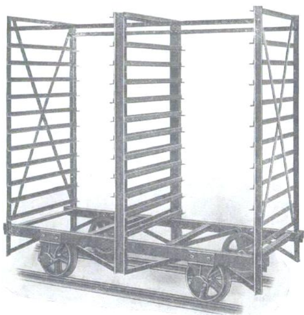
FIGURE 12. STEEL RACK CAR FOR TRANSPORTING BRICK ON PALLETS.
