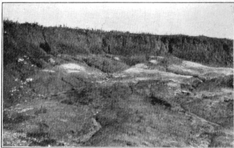
A. RESIDUAL CLAY AND LAFAYETTE OVERLYING SELMA CHALK, MACON.
