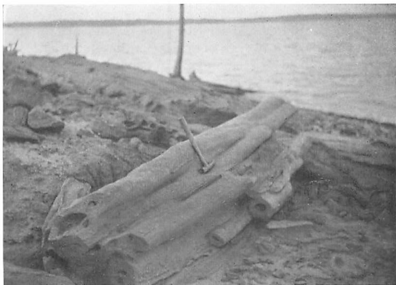
Figure 30.—Kosciusko pipe sandstone (Near Center, Sec.12, T.8 S., R.5 W.) at southeast end of Sardis Dam. October 19, 1954.
