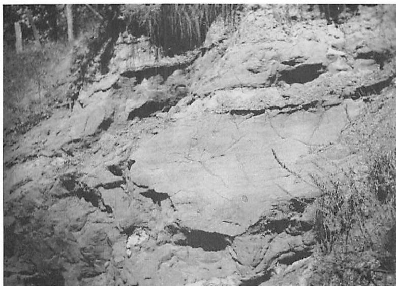
Figure 32. —Kosciusko-Citronelle contact (SW.Cor., Sec.28, T.7 S., R.6 W.) in the west wall of Clarendon Creek Valley 2 miles northwest of Sardis Dam. September 14, 1954.
