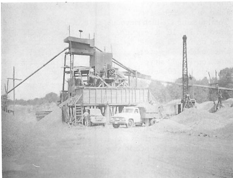
Figure 45.—Washing and screening plant. Crystal Springs Sand and Gravel Company (SW.¼, Sec.33, T.6 S., R.9 W.), 2 miles northeast of Crenshaw. July 28, 1953.
