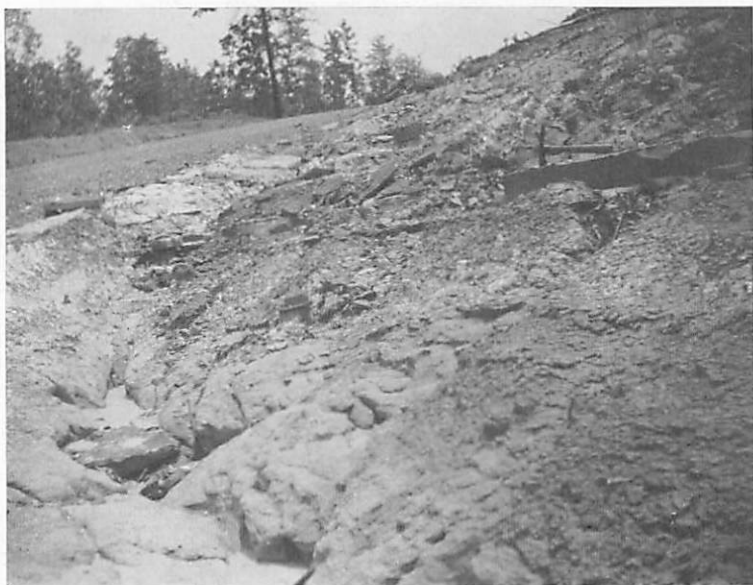
Figure 5. —Tallahatta-Kosciusko contact (E.part, Sec.33, T.9 S., R.5 W.) three quarters of a mile west of Sandy Springs Church, and a mile west of Orwood. June 9, 1955.
