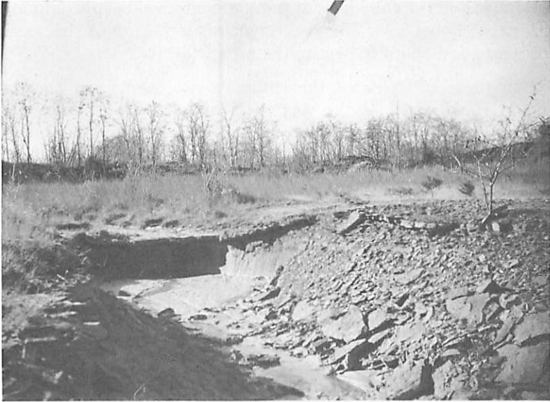
Figure 22.—Top of Zilpha formation (SW.Cor., Sec.12, T.8 S., R.5 W.) a quarter of a mile south of Sardis Dam spillway. December 10, 1952.
