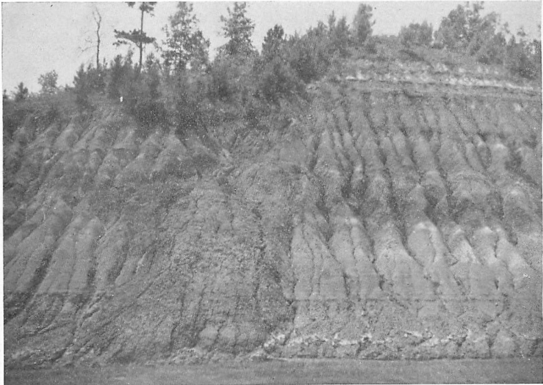
Figure 4.—Tuscaloosa clays exposed by U. S. Highway 78 cut (NE. 1/4, Sec. 6, T. 10 S., R. 10 E.) in the west wall of Gum Creek Valley 7.5 miles east-southeast from Fulton. September 7, 1945.
