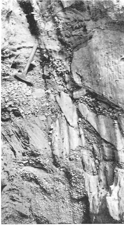
Figure 18.—Angular sand and silt blocks in a sand and gravel matrix. East face of Wm. G. Walter gravel pit, one mile south of Morton. August 31, 1941.
