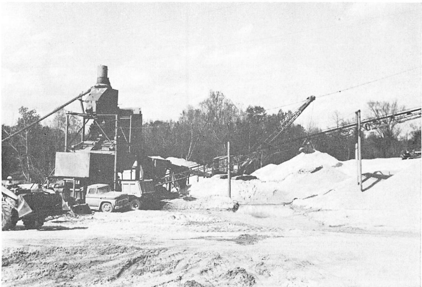
Figure 21.—Separator at gravel washing plant. Perry Nations photo. April 22, 1966.
