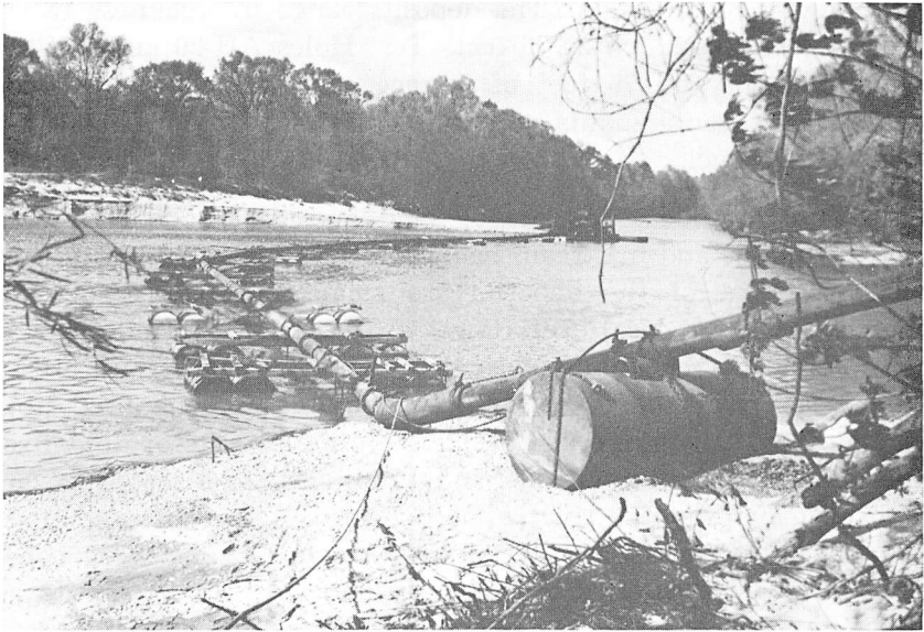
Figure 20.—Dredging barge at gravel washing operations on Bayou Pierre near center of NW. \frac{1}{4} of irregular Sec.24, T.12N., R.4E. Perry Nations photo. April 22, 1966.
