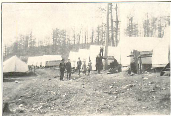
View of Camp of Memphis Mining and M'fg. Co., on Reid property, Potts Camp.
