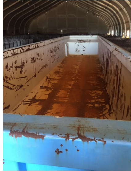
Mix Box located within IB Structure
