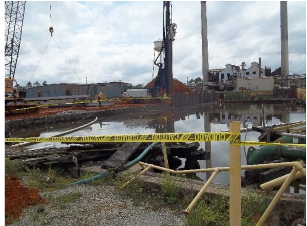
Sheet piles being advanced by ABI machine
