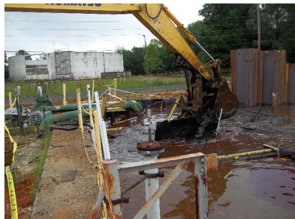
Removal of IB baffles on east end of IB
