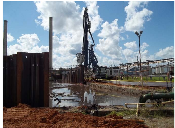
Sheet pile installation
