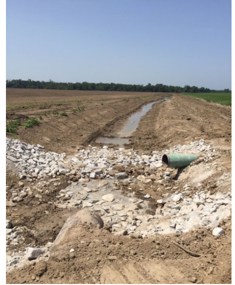
Two stage Ditch Low Grade Weir
