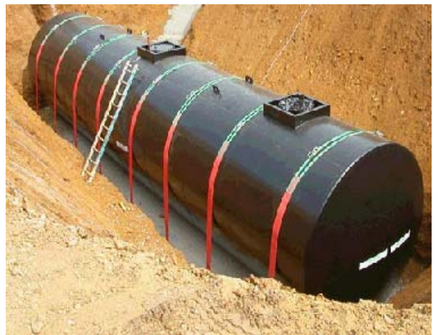
Underground storage tank installation
