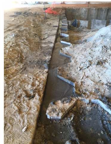
Annular ring after flowable fill placement
