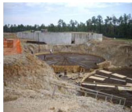
Texas Flat Waste Water Treatment Facility in Hancock County
