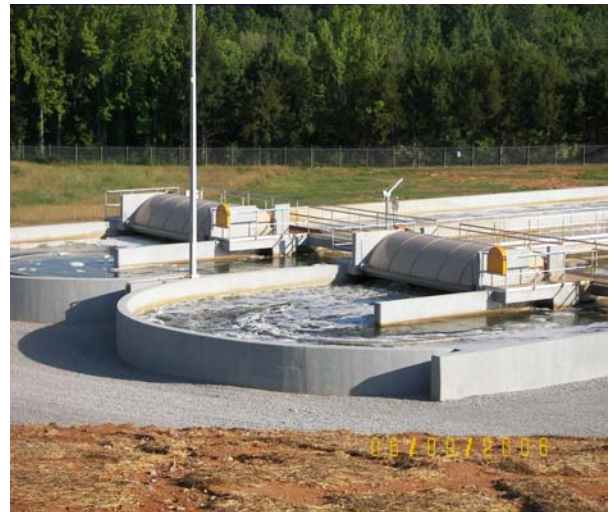
Pontotoc Wastewater Treatment Plant
