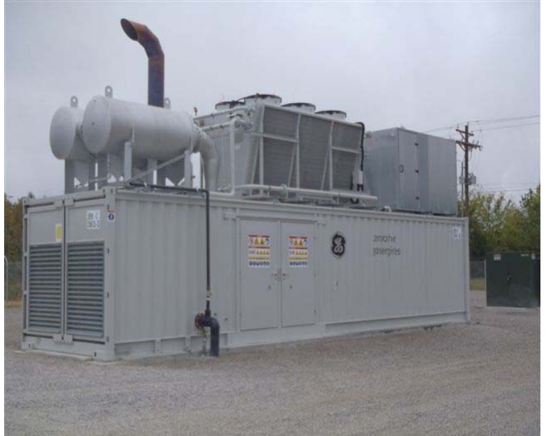
Mississippi's first landfill gas to electricity generating facility at the Golden Triangle Landfill
