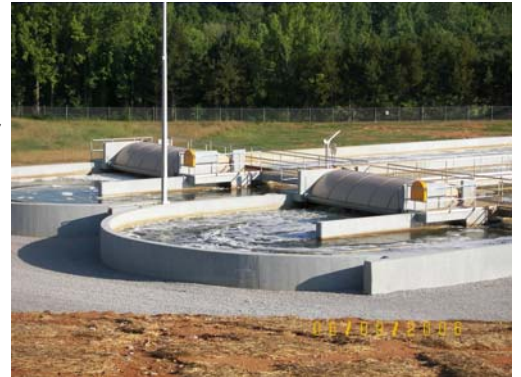
Pontotoc Wastewater Treatment Plant
