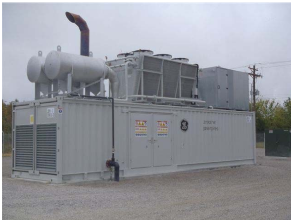
Mississippi's first landfill gas to electricity generating facility at the Golden Triangle Landfill
