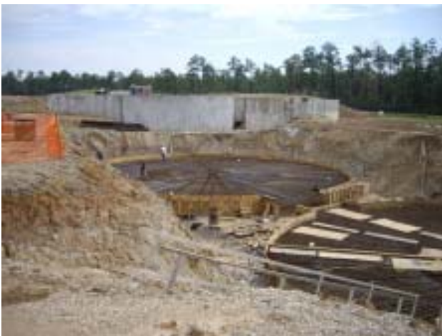
Texas Flat Waste Water Treatment Facility in Hancock County
