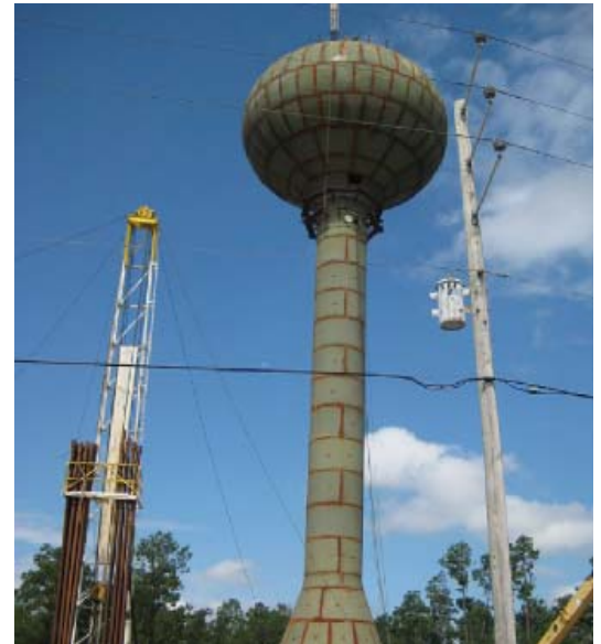
Stone County Ten Mile Road water project
