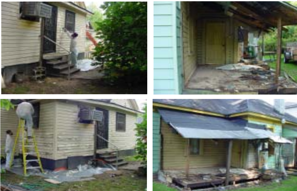
Lead-based paint inspection and removal.
