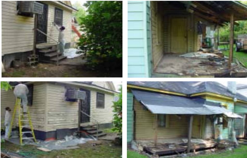
Lead-based paint inspection and removal.
