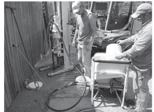
Hydrogen Release Compound is being injected to remediate a dry cleaner on the Gulf Coast
