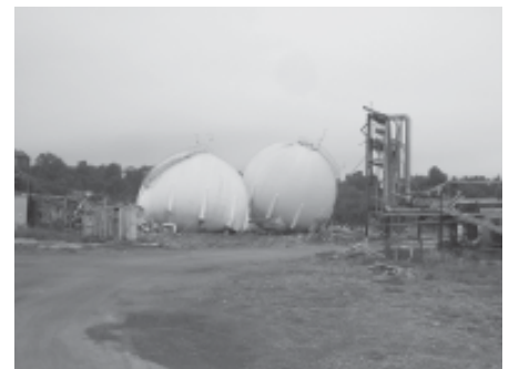
Demolition Work at Abandoned Vicksburg Chemical Plant
