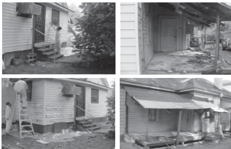
Lead-based paint inspection and removal.
