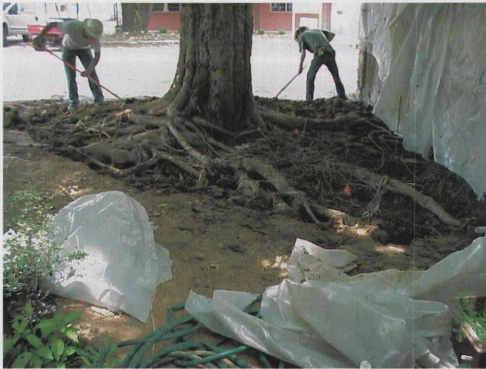
Photo 7 – Remediation crew spreading clean backfill over exposed tree roots following completion of the root washing process. Note the red flags marking confirmation-sampling locations within the root zone.
