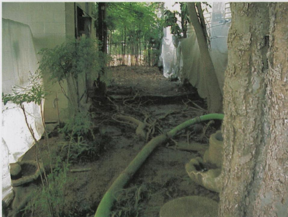
Photo 8 – View looking south between the Garment Shop building and the Kellum house showing exposed tree roots following removal of impacted soil using the “AirShovel®”. The hose shown in the foreground is the vacuum hose used to remove the soil and water slurry.
