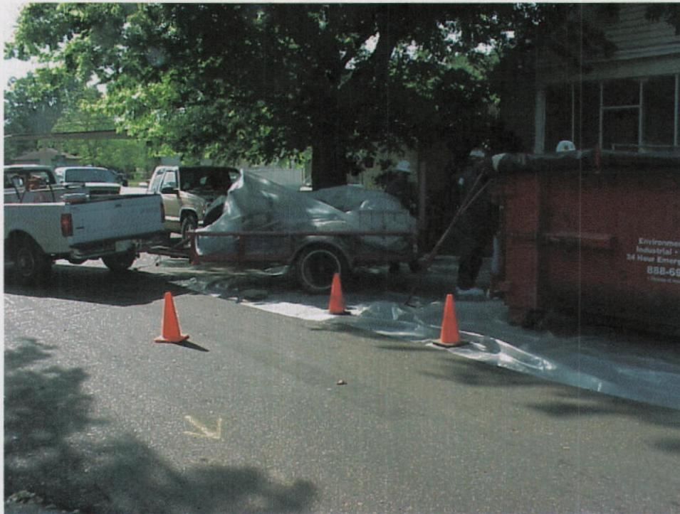
Photo 3 – Yard furniture and other non-porous articles are being removed to the decontamination pad on the Kuhlman property for cleaning. The plastic covering prevents dust from blowing off of the articles.
