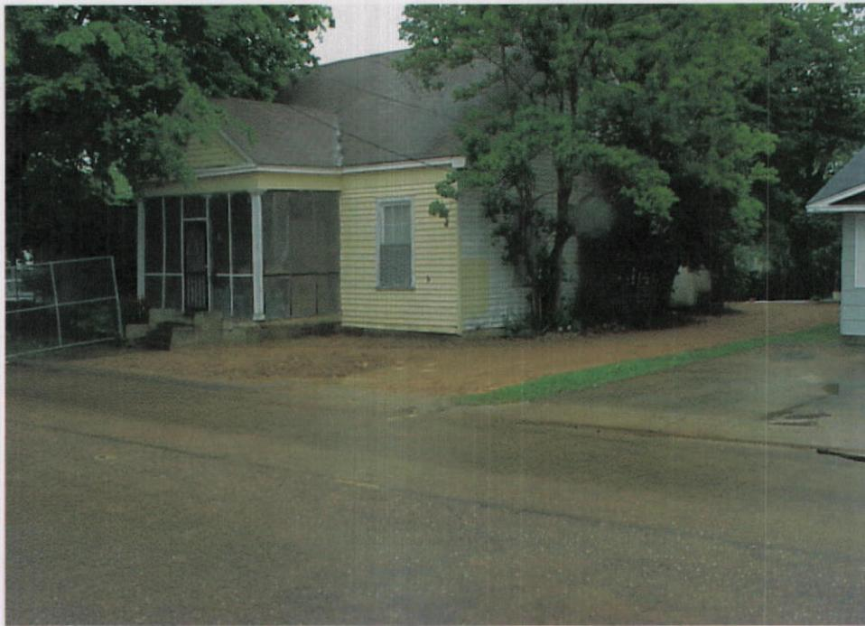
Photo 9 – View of the Kellum house and yard after removal of impacted soil and placement of clean back fill. The area behind the temporary fence on the left side of the photo and the area with trees beside the driveway are awaiting root washing.
