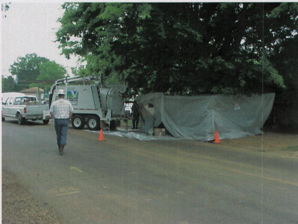
Photo 6 – Cleaning of the hackberry tree roots. The “AirShovel®” unit is shown at the left of the photo. The plastic sheeting is used to cover the work area to provide security and eliminate splashing of water and soil outside the work area.
