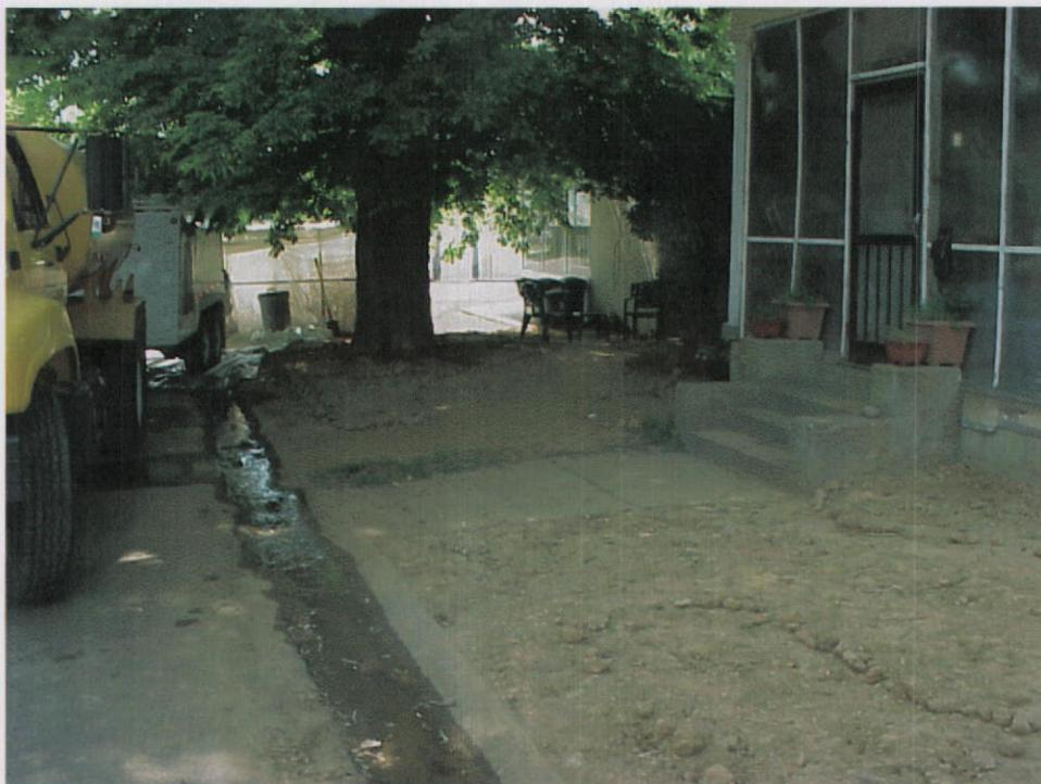
Photo 10 – View of the Kellum front yard looking east following removal of impacted soil and placement of clean soil. Planting areas are marked off on the ground with stones awaiting shrubs and bedding plants.
