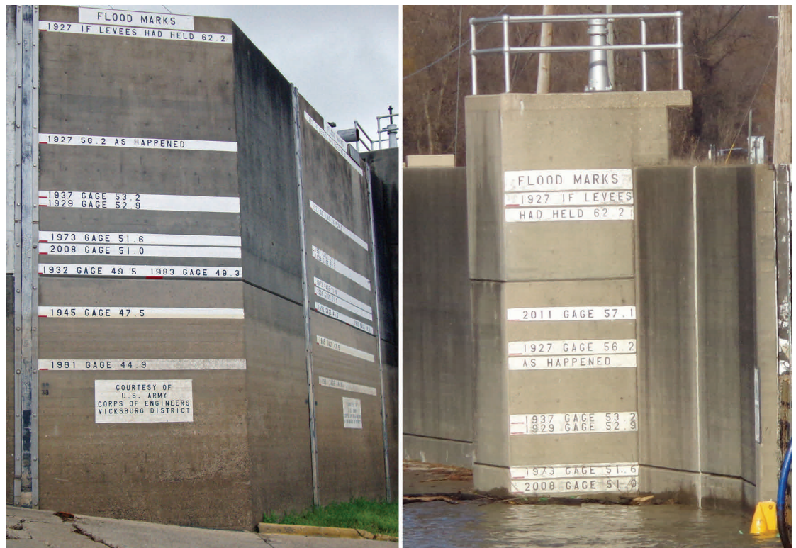
Figure 2. Left, Flood crests recorded on the flood wall at Vicksburg after the flood of 2008; picture taken on September 26, 2009. Right, Flood level a day before the crest as seen against the Vicksburg flood wall on January 14, 2016.
