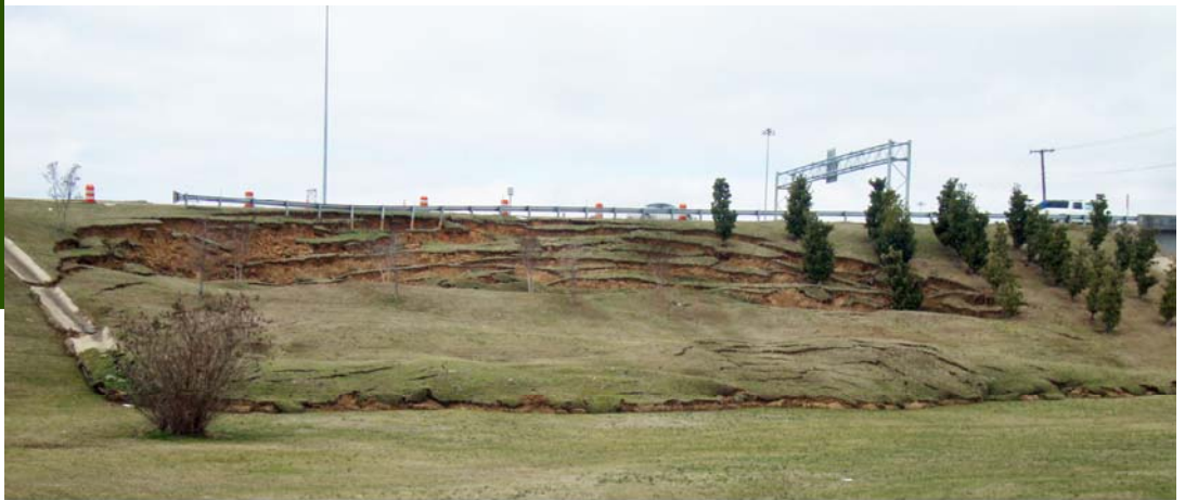
Figure 1. Slump in Yazoo Clay on Interstate 220 North just south of Highway 80 in Jackson. Picture was taken on February 27, 2015.
