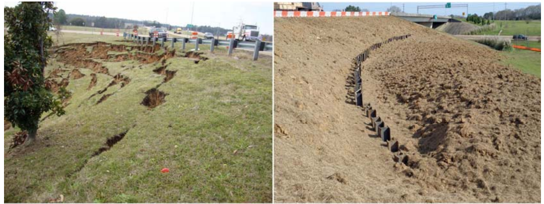
Figure 3. Left, looking south at slump in Yazoo Clay on Interstate 220 North at Highway 80 in Jackson on February 27, 2015. Right, looking north at slump after repairs on March 17, 2015.
