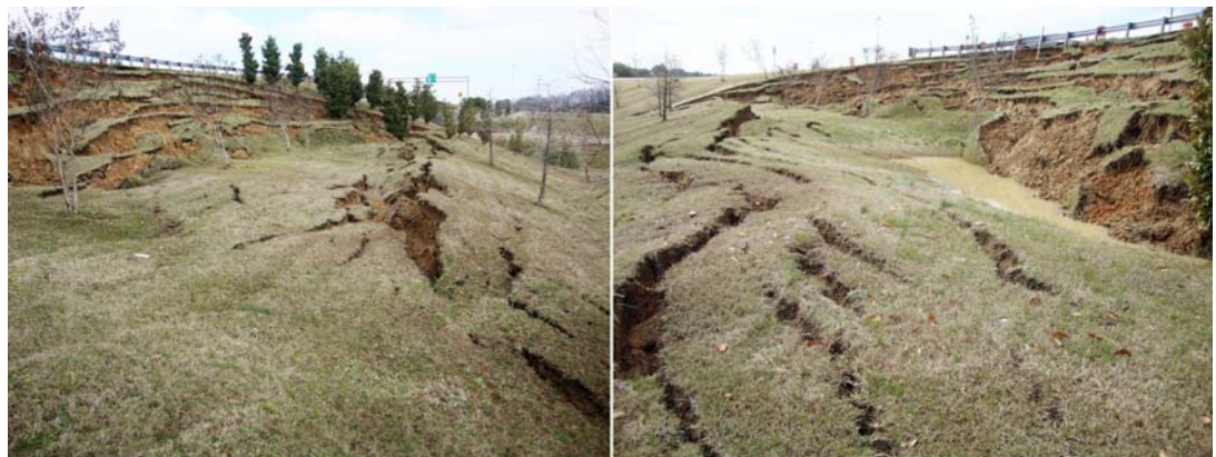
Figure 2. Left, looking north at slump in Yazoo Clay on Interstate 220 North just south of Highway 80 in Jackson. Right, looking south at slump. Pictures were taken on February 27, 2015.
