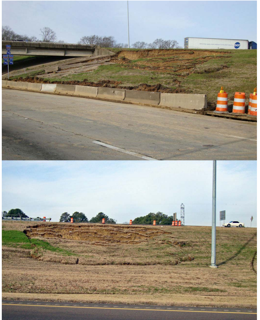
Figure 6. Top, slump in Yazoo Clay on Terry Road at Interstate 20 in Jackson. Bottom, slump in Yazoo Clay on the east side of Interstate 220 North near the I-20 interchange. Pictures were taken on February 10, 2010.
