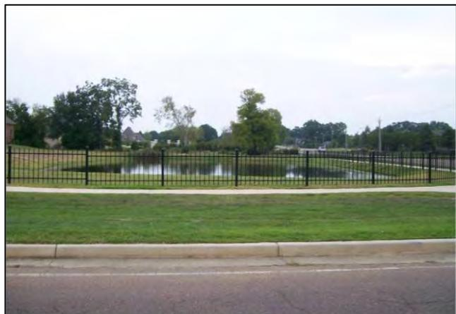
Fencing of wet detention basins is not generally aesthetically pleasing but may be required by the local review authority. A preferred method is to engineer the contours of the wet detention basin to eliminate drop-offs and other safety hazards as discussed above. Riser openings must not permit unauthorized access. End walls above pipe outfalls greater than 48 inches in diameter should be fenced to prevent falls.
