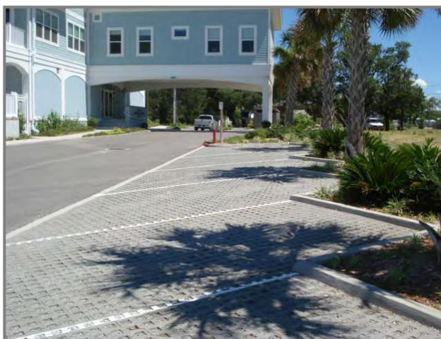
Specific design requirements relating to the structural stability of permeable pavements are beyond the scope of this manual. The reader is referred to the AASHTO Flexible Pavement Method for structural design requirements. The following guidelines are presented to ensure that permeable pavements are properly located, designed, and constructed to meet water quality objectives.
