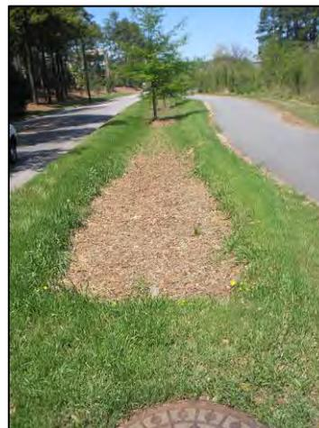
Figure 3 shows a bioretention cell with a pretreatment forebay. Notice the sediment that has settled onto the rocks. Without the forebay, this sediment would have collected on the top of the bioretention cell, clogged the soil media, and would have become a maintenance burden. Forebays that are located inside a cell should be lined in order to ensure that the treatment volume drains through the media.
