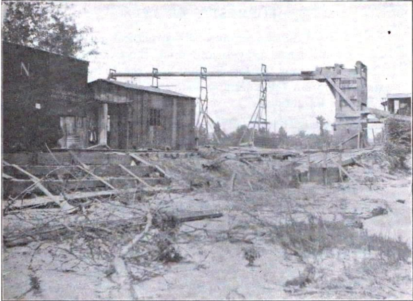
PLATE VIa.—Screen of the Louisiana Sand and Gravel Company, near Hattiesburg
