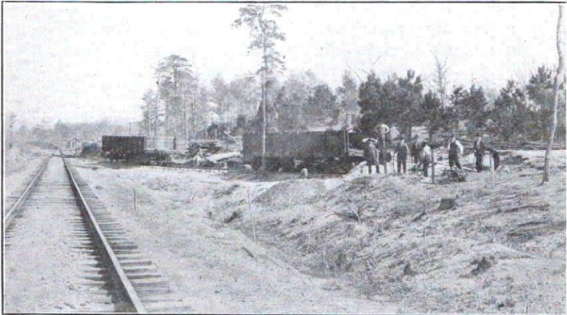
PLATE XIII.—Opening of the Tishomingo City Gravel Pit. Gravel at Right of Car near Which the Men are Standing.
