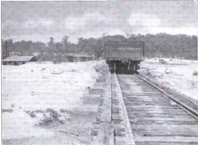
PLATE VIb.—General View of the Louisiana Sand and Gravel Company's Plant, Hattiesburg.
