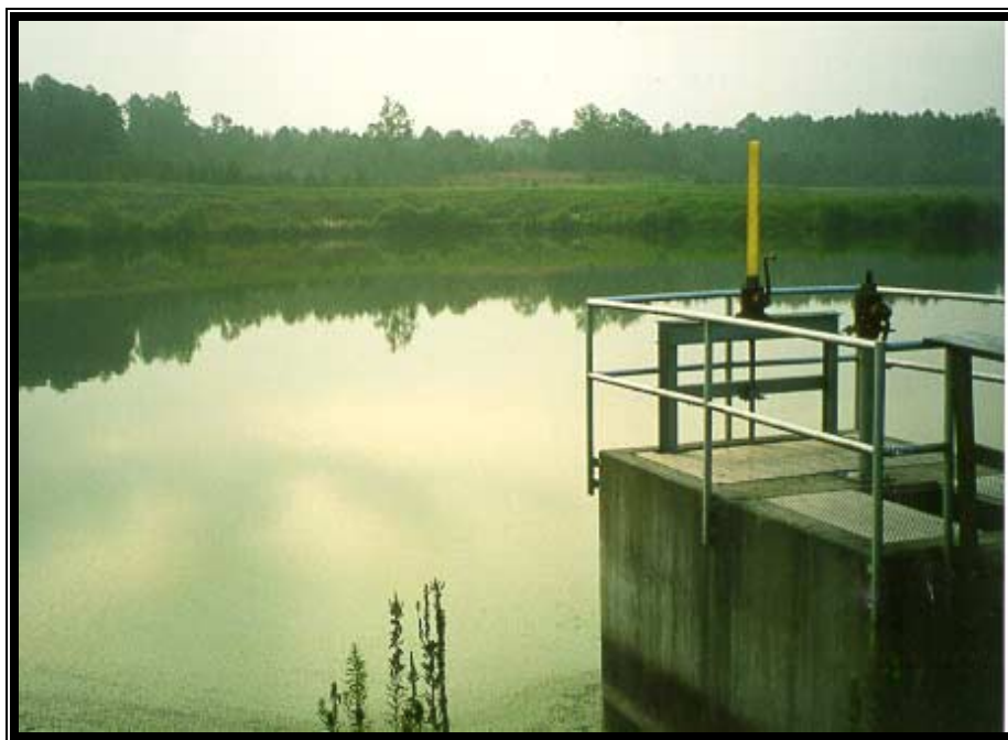
Photo 4. Iuka POTW Facility, Second Cell
